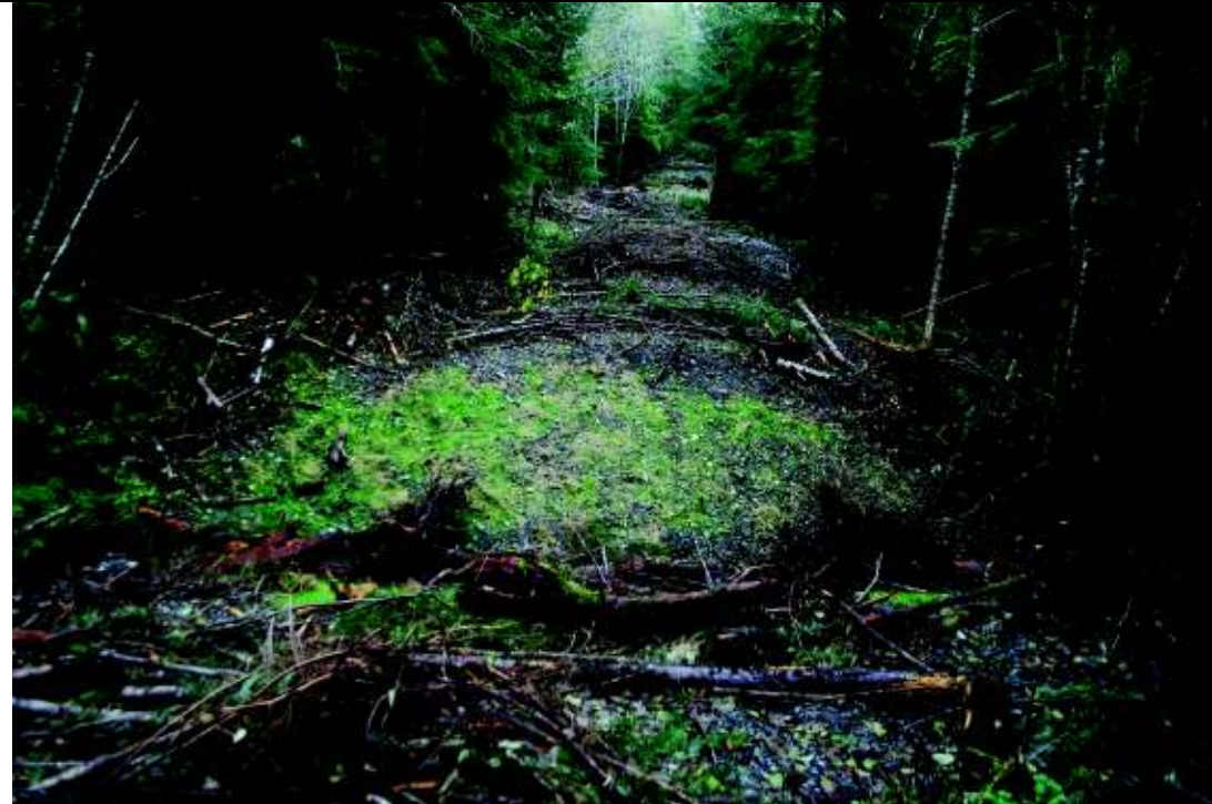
Photo 5. Decommissioned upper Pole Creek Basin road, including woody-debris placement.
