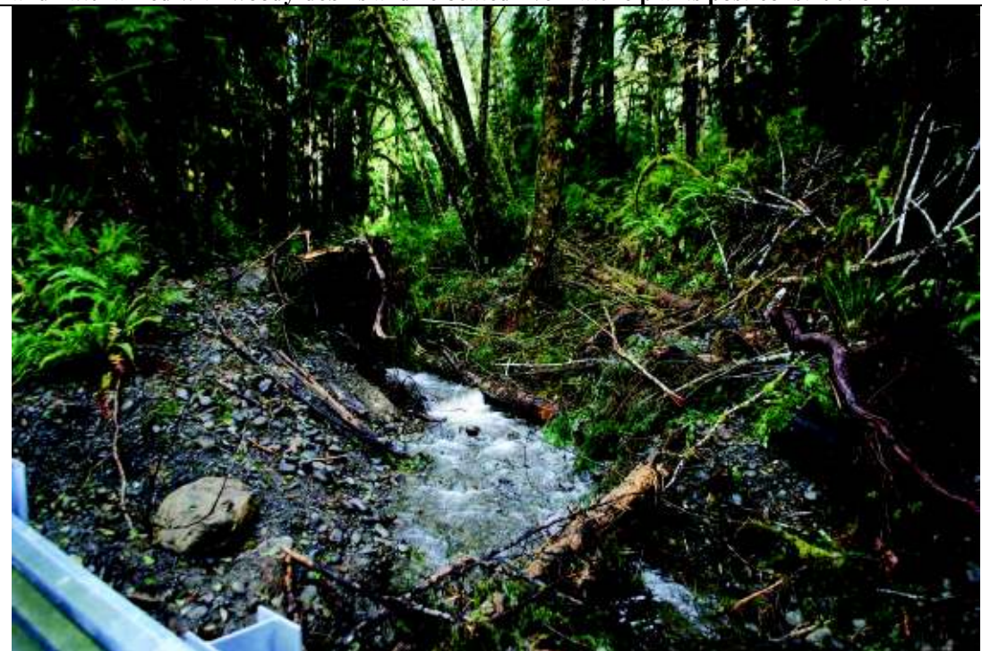
Photo 4. Pole Creek conditions upstream of new bridge, including woody-debris in stream, and naturalized construction area
