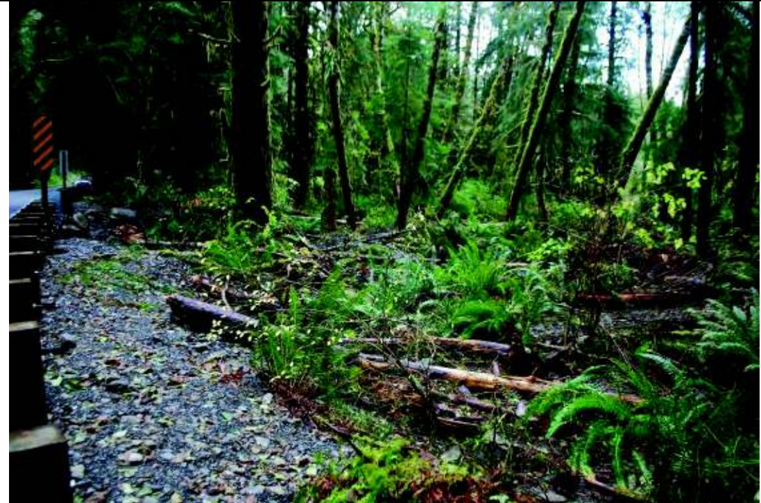
Photo 1. Site of Upper Hoh Road bypass used during bridge construction and decommissioned and naturalized with woody-debris and relocated live mature plants post-construction.
